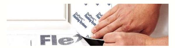
**DuPont™ Flashing Tape** helps protect the heads and jambs of rectangular doors and windows from air and water intrusion.
