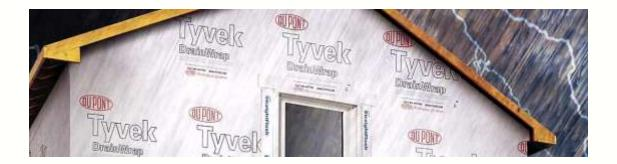
**DuPont™ Tyvek® DrainWrap™** is a moisture barrier designed to provide enhanced drainage in areas subject to extreme, wind driven rain.
