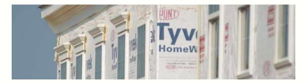
**DuPont™** 9 x 150 Tyvek® HomeWrap® is the original house wrap, incorporating unique material science that helps keep air and water out, while letting water vapor escape.
